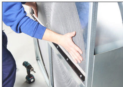
(8) Incline the warming wheel carefully. Be careful not to damage the delicate storage mass
