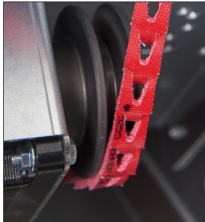
When fitting the drive belt, pay attention to the direction of rotation of the storage mass. The running direction is marked on the belt elements by an arrow
