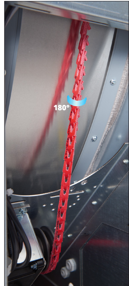
After a few revolutions of the storage mass, the drive belt twists once in such a way that the locking pins turn outwards
