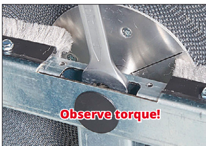
(10) Once the heat wheel has been set to the appropriate inclination, the position is fixed by tightening the hexagon head screw (for torque, see Tab. 2)
