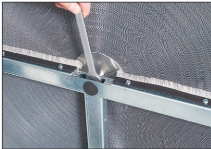
(7) Loosen the hexagon head screw
