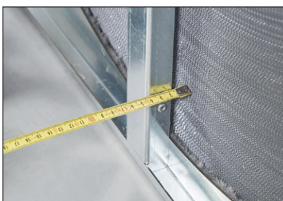
(11) Check the centring of the heat wheel in the vertical centre of the housing, measuring points see (9) on both sides.
