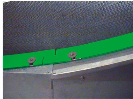
Permanently fixed plastic seals or profiled sheet metal with extremely small clearance to the rotor are used as center seals.
